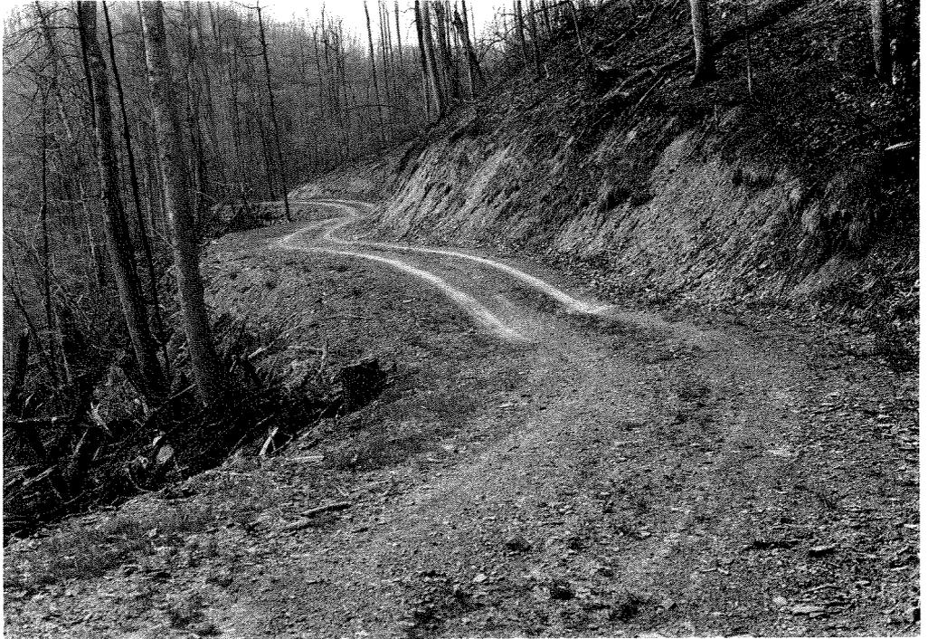
Figure 2.-A minimum-standard road showing a broad-based dip in the foreground.
